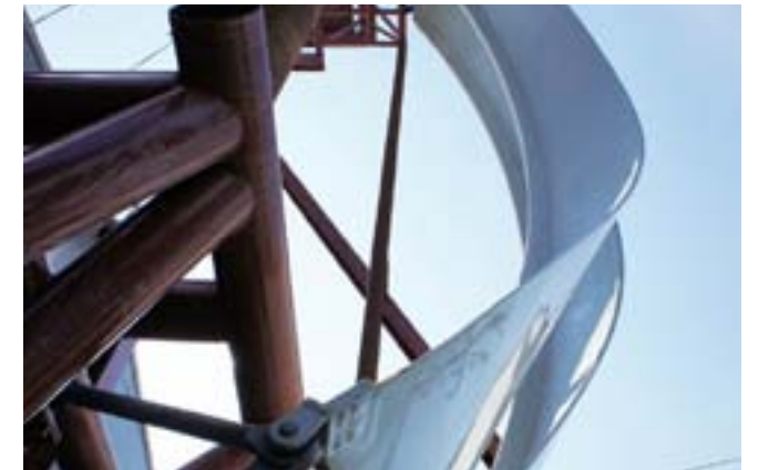
5 13 meter GFRP Prototype of gill like adaptive shading of Ocean One, SOMA
